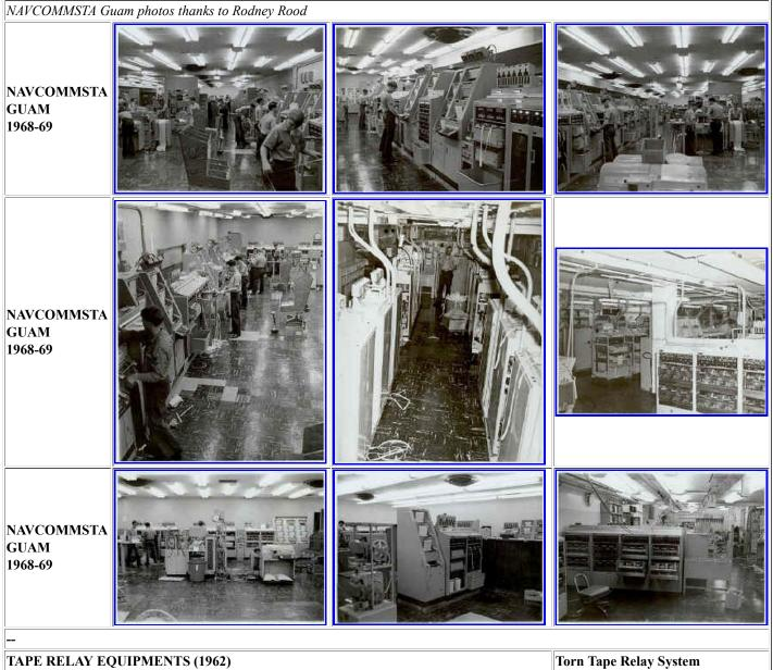
The volume of teletypewriter traffic relayed by NAVCOMMSTAs and many of the smaller shore stations has led to the development of tape relay equipment that requires a minimum of operator attention. In figure 1 below are receiving banks or console packages, which house several typing reperforators for use on incoming lines in torn-tape relay centers. The operator logs each
