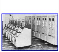
If duplicate copies of relayed traffic are required for the files, monitoring equipment (not shown in fig. 7-32) is used. This is a group of typing reperforators which produces duplicates of tapes undergoing transmission on the sending bank, and winds the monitor tapes on reels suitable for stowage. The monitoring equipment also duplicates the channel number for each message, providing a means of reference should the message be needed in the future.
